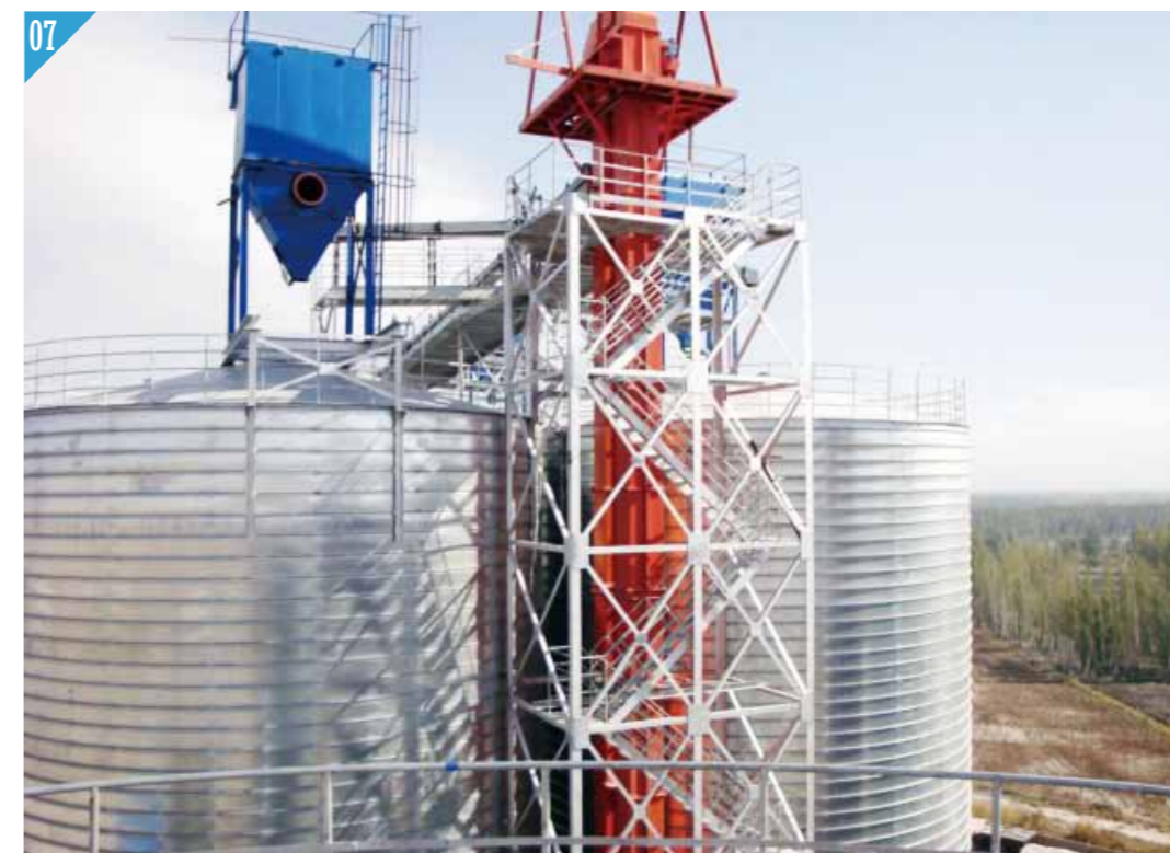
Auxiliary Equipment Installation
