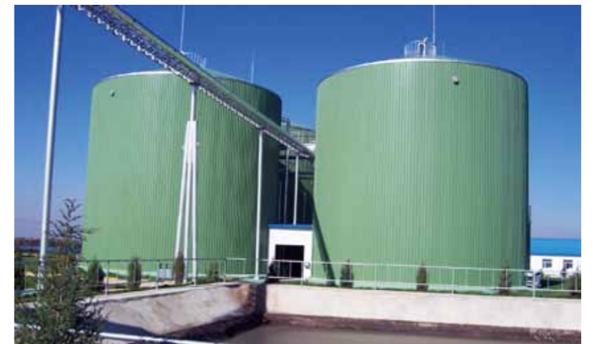
Pingdingshan Sludge Treatment and Disposal Project
